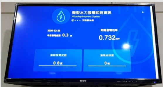
Plant site monitoring system screen display
